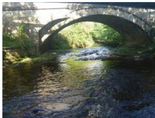
The newer structure built over an earlier bridge from Artlebeck
